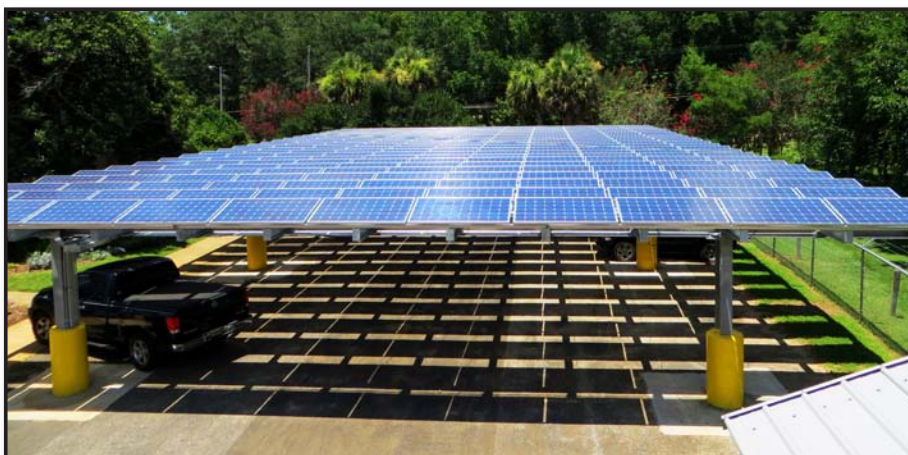
Leon County Net-Zero Facility
